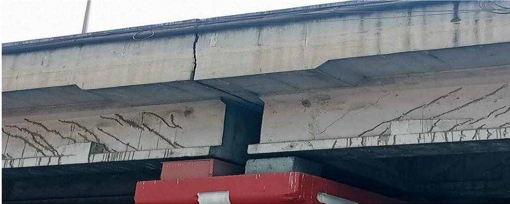
**Fig. no.3** Cracks Developed On Psg Girder At Hadapsar, Pune, Maharashtra Bridge. Due To Excessive Loading And Design Failure.
